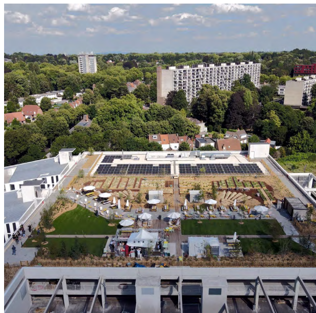
Nhood Services France, Le Compact_2
